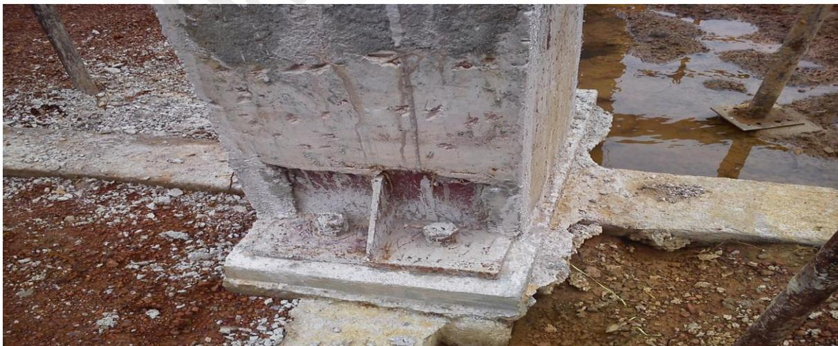
*Steel column bolted to foundation cap and covered with a coat of concrete*
